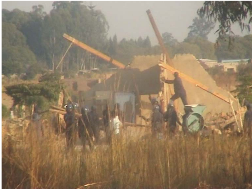
Fig. 1. Police supervised destruction of illegal structures
